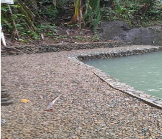
Figure 9: Maintenance and gravelling of the upper pool.
